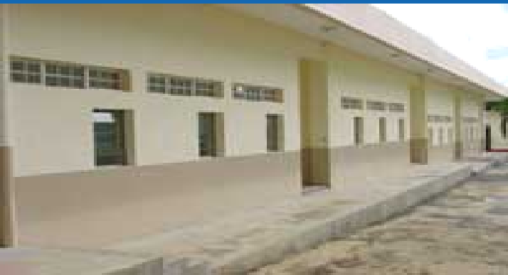
Queen Victoria School Renovation
